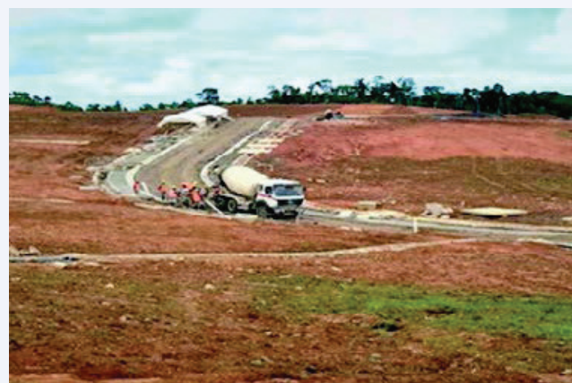
Work in progress at Davuilevu site.
